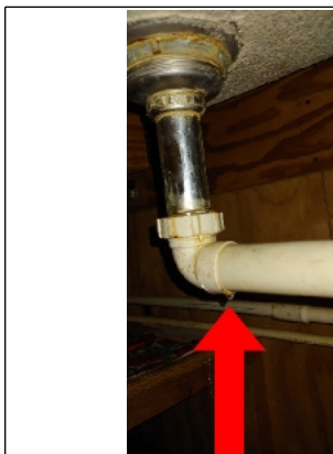
Leak underneath kitchen sink. Recommend repair.
