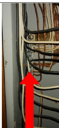
Neutrals and grounds should be on its own separate busbar for proper grounding. Double-tapping observed. Repairs needed.
