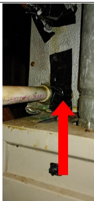
Recommend adding a PVC pipe with float switch / kill switch in case main drain gets clogged.
