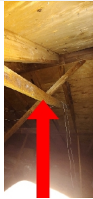
Sagging collar ties throughout attic. Recommended structural engineer.
