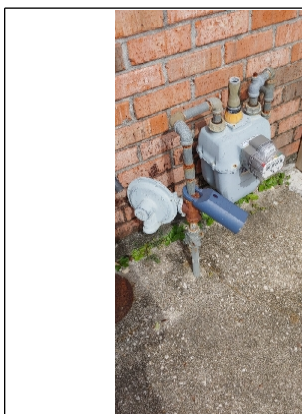
Fuel shut off valve location. Information for a future homeowner.
