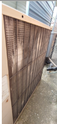
Exterior AC fins are damaged. Recommend reevaluated by license HVAC technician.
