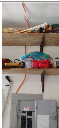
Substandard wiring.
