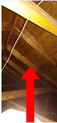
Improper installed sister board repairs. Recommended structural engineer.
