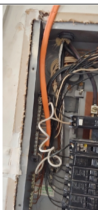
Substandard wiring.
