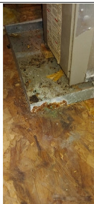
Deterioration observed on condensation pan and moisture staining observe. Recommend reevaluated by license HVAC technician.
