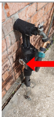
Secondary water shut off valve location. Information for a future homeowner.
