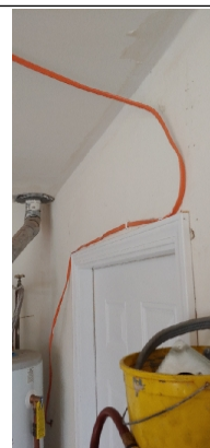
Substandard wiring.
