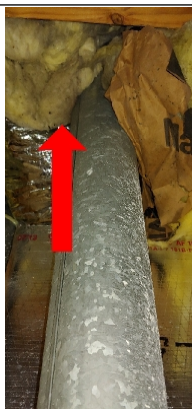
Gas B vents recommend a 1 inch clearance from combustibles.
