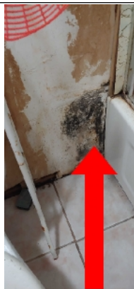
Possible mold or mildew. Recommend tested. Potential safety hazard.
