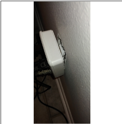
Missing electrical cover plate. Potential safety hazard.
