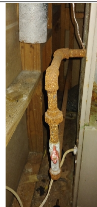
Rusted gas piping. Recommend reevaluated by license HVAC technician.
