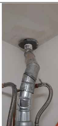
B vent is not secure properly, different size connections, and loose metal thimble up top. Possible carbon monoxide leakage. Potential safety hazard.
